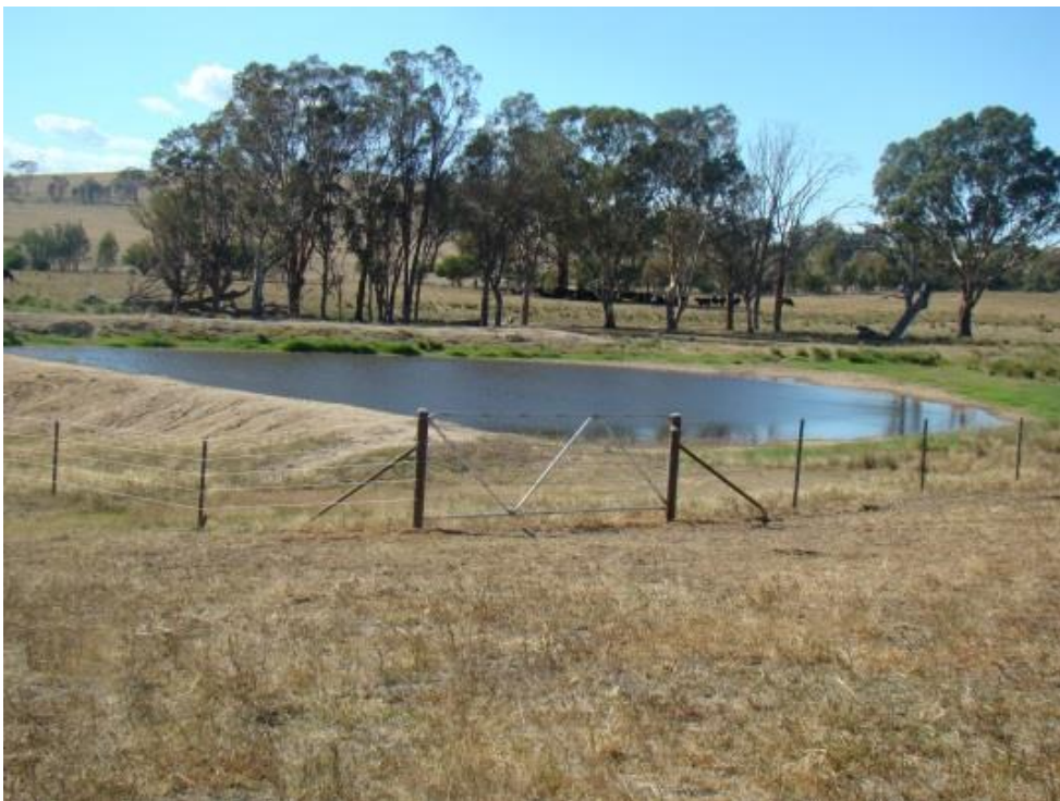
The dam: in May 2014, prior to any work (top) and in March 2015, fully fenced (bottom)
