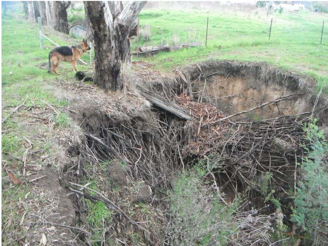
Figure 4: Site 4, Headcut on Dellhaven.
