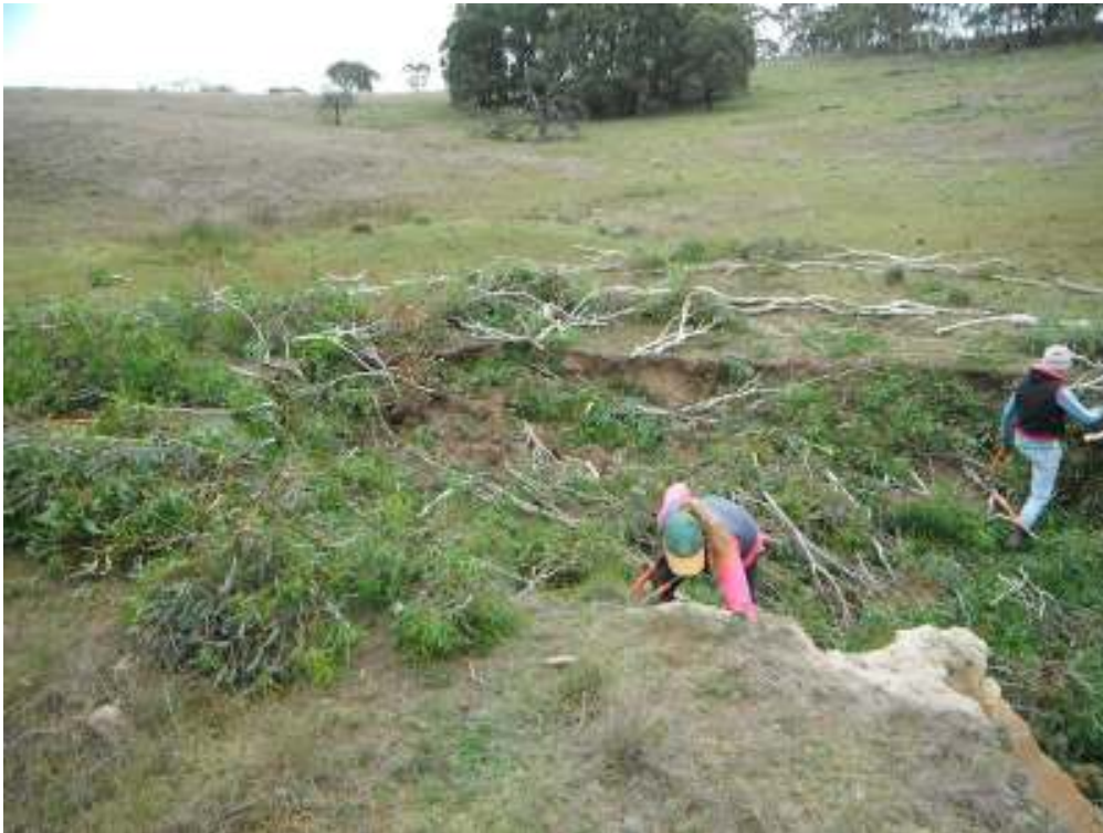
Figure F1: Brush is laid across the battered face, butt end upstream, working uphill. While battering, soil and brush laid in alternating layers helps to reinforce the soil.
