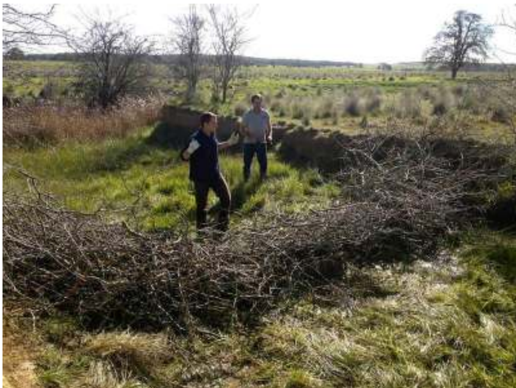
Figure C3: Brush in place ready for stomping down and wiring to the logs. The brush is laid in alternating directions and overlapped to ensure it binds together well. Any material can be used, but prickly material like this Hawthorn binds together particularly well.
