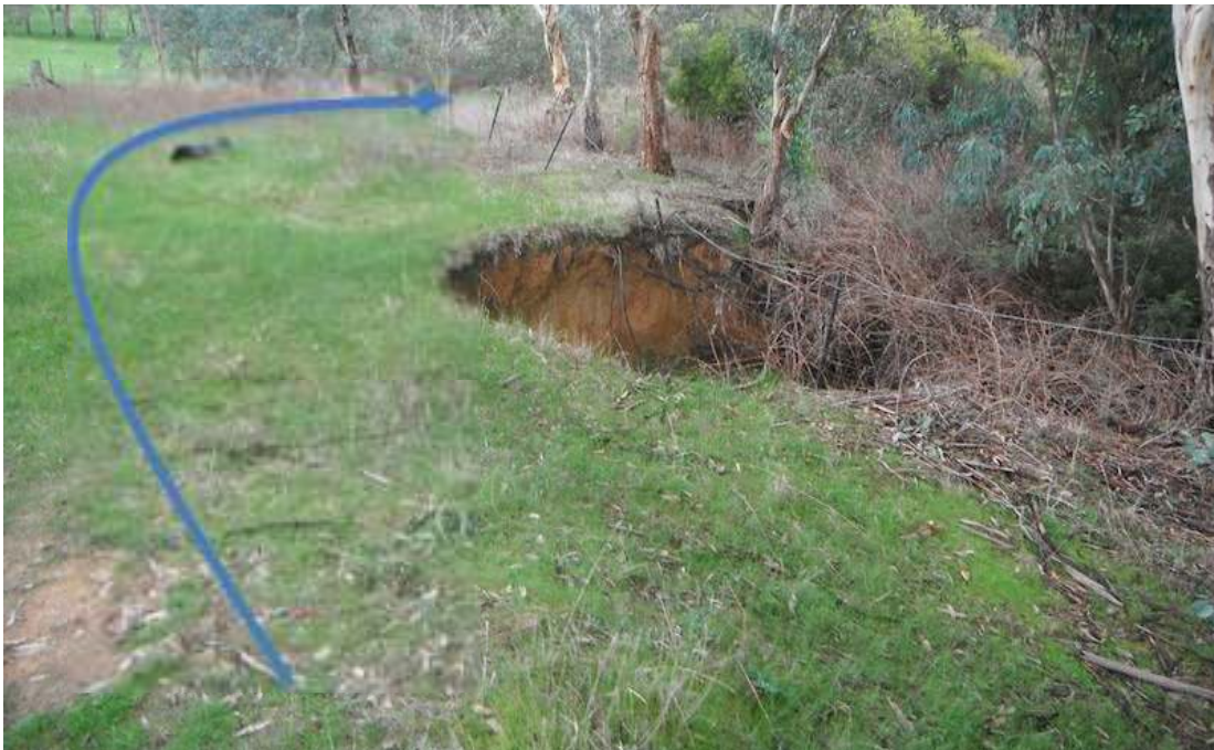
Figure 3.2: Potential flow diversion path. Shrubs seen in the background, planted on by the owners of Waddon would be threatened if another headcut commenced as a result of the new flow path.
