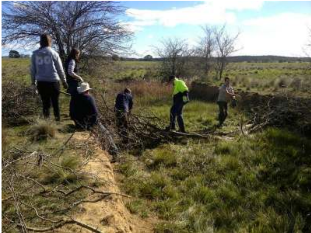
Figure C2: Brush laying commences following the securing of the logs.
