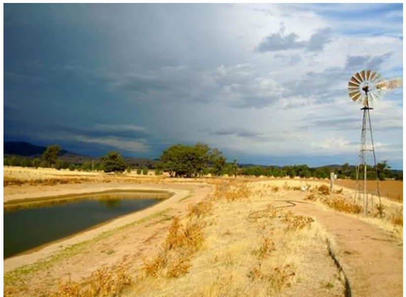
The dam in summer 2014, prior to any work; remnant vegetation can be seen just beyond the dam
