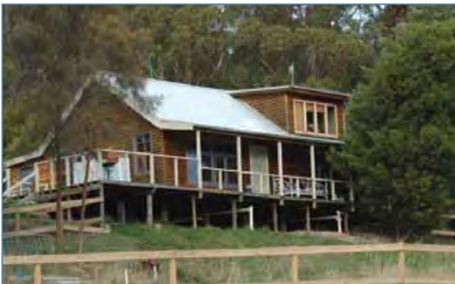
Figure 19. Pier or post style construction has considerably lower risk of initiating tunnel erosion than cut and fill techniques.
