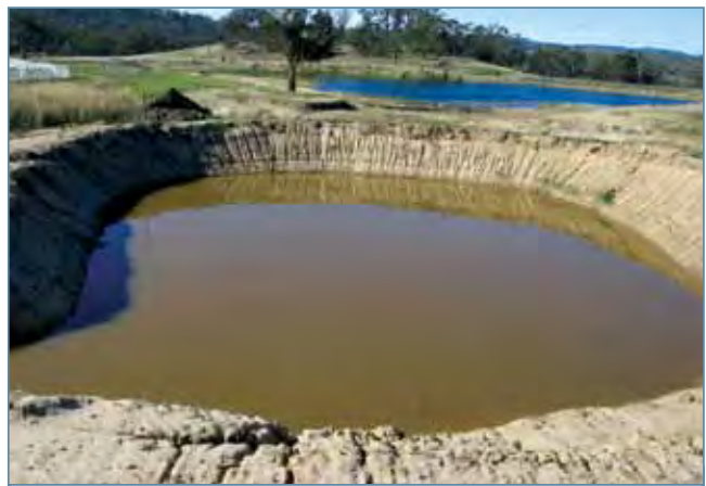
Figure 32. The dam in the foreground has been constructed from dispersive clays. Note the rill erosion and cloudy brown colour of water in foreground, compared to the blue colour of the dam constructed from non-dispersive soils in the background.
