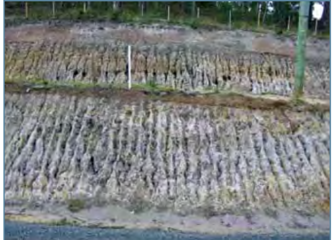
Figure 28. Rill and tunnel erosion caused by excavation of sodic soils for road construction. Dunalley.
