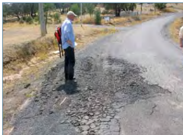
Figure 25. Road surface breaking up due to construction on dispersive clays. This section of road is repaired 2-3 times a year.
