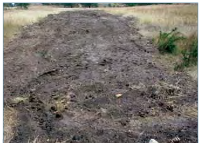
Figure 37. Good technique. Topsoil mounding, reclaimed tunnel erosion, Brighton. Note the width of earthworks required to fix a 50cm wide tunnel, and the raised profile to shed surface water. Jute cloth would prevent surface erosion until vegetation has established.
