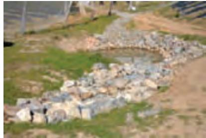
A sediment pond at the farm's lowest point allows this plantation to discharge cleaner water.
