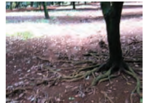
Exposed tree roots
