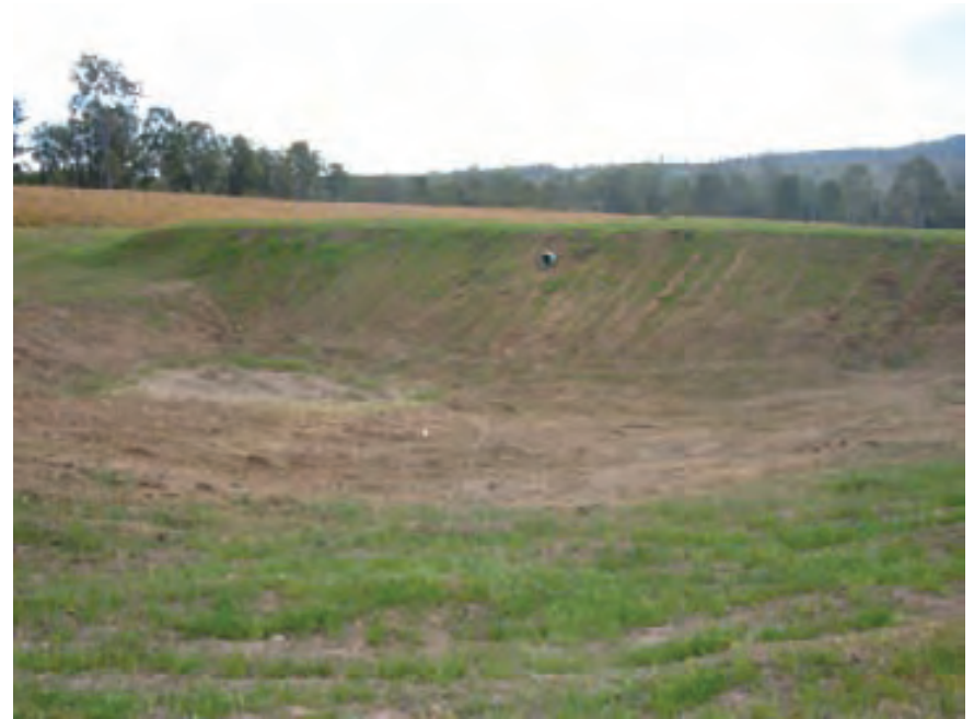
A newly constructed gully dam, showing the excavation, embankment, spillway and a trickle pipe for low flows.
