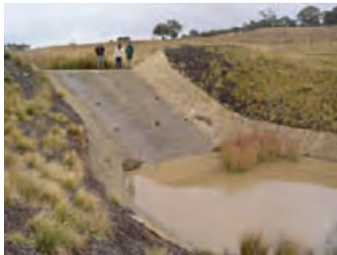
A concrete drop structure
