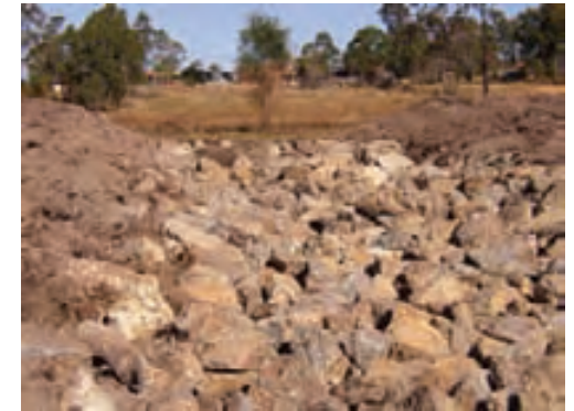
Rock drop structure with earth guide walls
