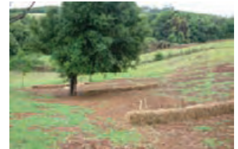
Hay bale check structures
