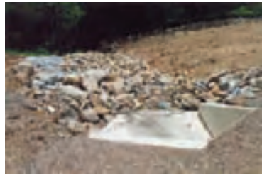
Rock protects the batter where this culvert emerges. Source: Tim Duckett IECA
