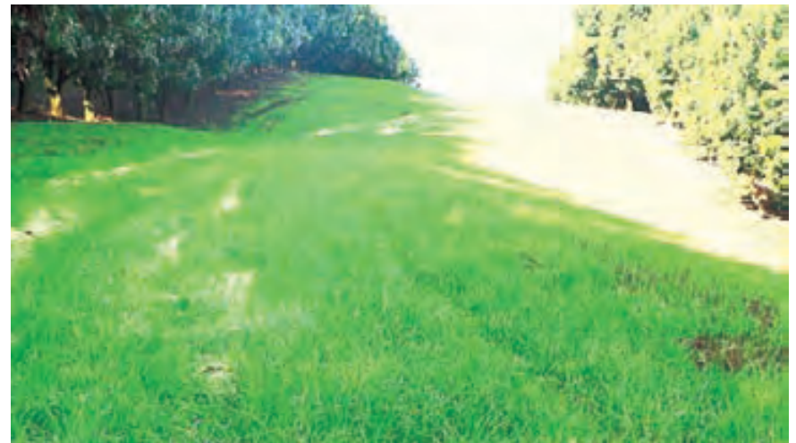
A diversion bank stops water from the upslope orchard from causing erosion in the block below. Source: Ian Clapham
