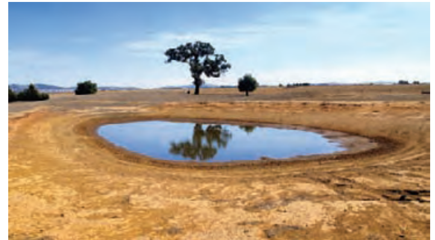
Excavated tank Source: Graham Johnson NSW DPI
