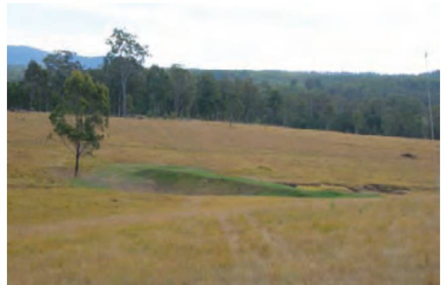
A gully control dam
