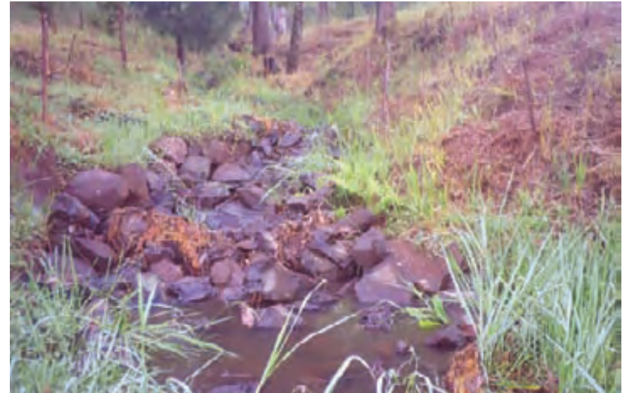
Protect persistently scouring channels with rock.
