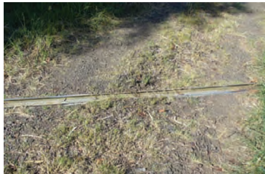
A recessed pipe set into a steep gravel track.
