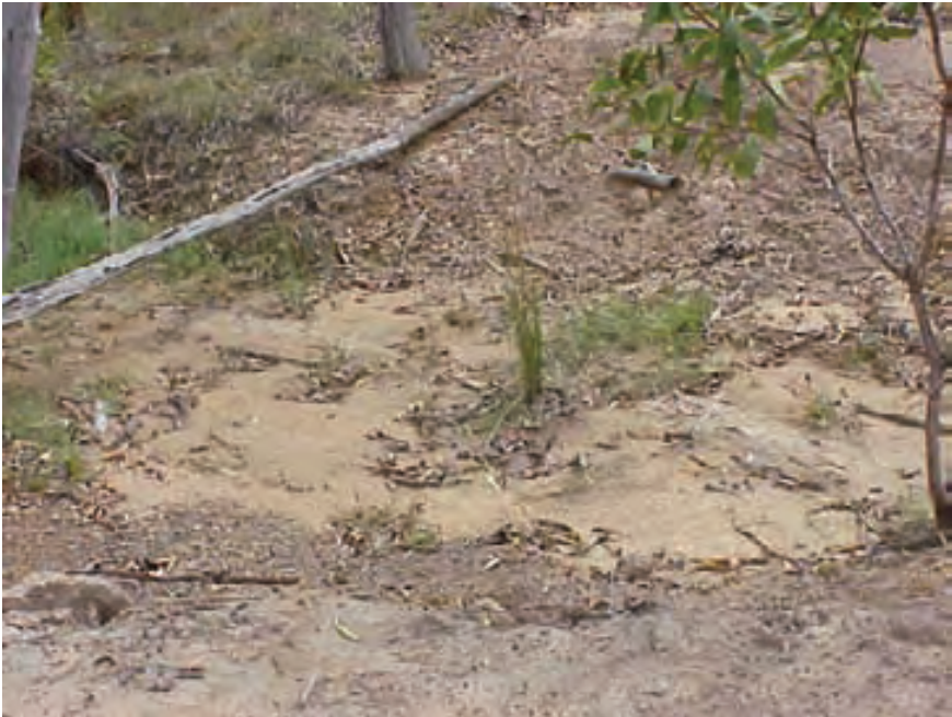
A sediment fan at the outlet of a tunnel.
