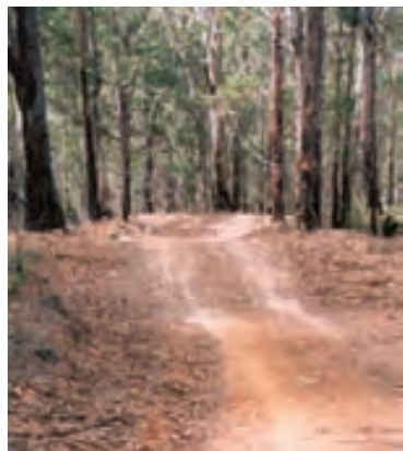
A cross bank stops water running down the track slope. Source: Michael Frankcombe IECA
