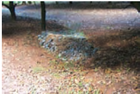
A small rock check structure
