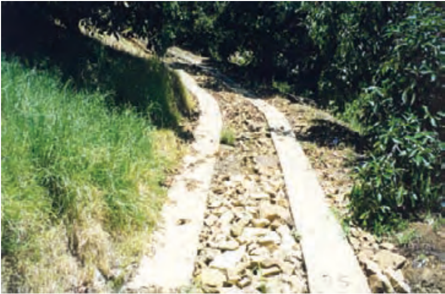
Concrete can be used to stabilise steep, high use tracks.
