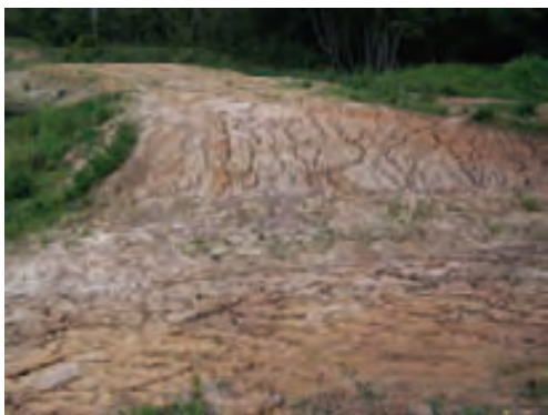
Rill erosion Source: Terrence Hudson
