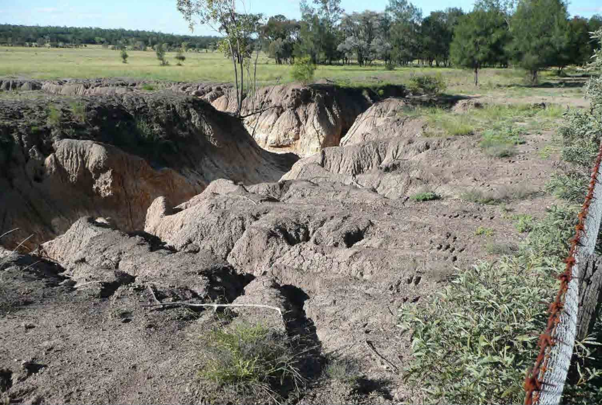
Gully erosion resulting from a failed diversion bank on a dispersive soil near Meandarra (150 km west of Dalby)
