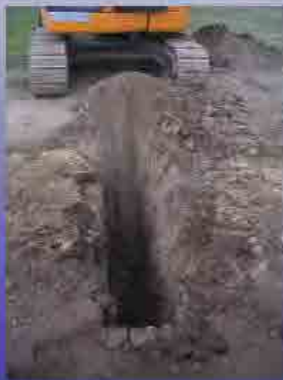
Excavate across trench/tunnel
