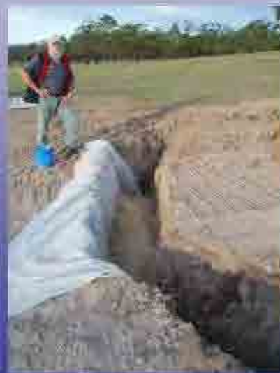
Geotextile downslope wall
