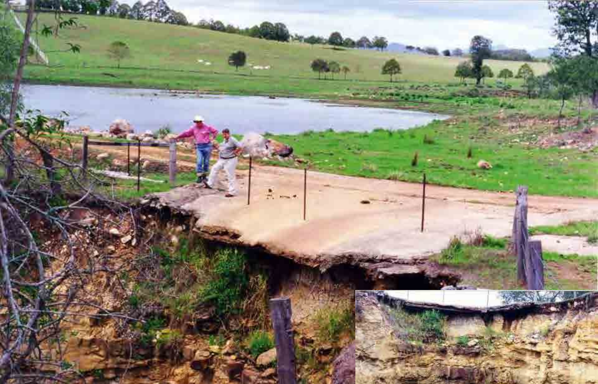
A 6 m high overfall in a dam bywash in dispersive soils in south-east Queensland. The concrete floodway is under threat and is the main entry to the property.
