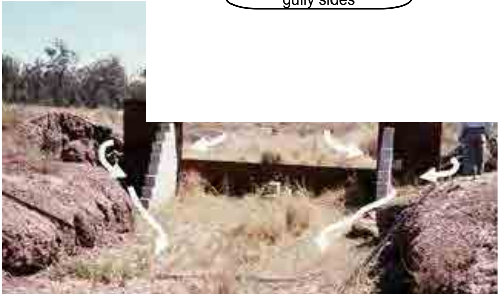
Bed stabilisation structure keyed into gully sides
