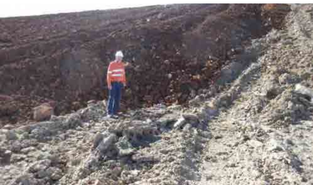
Adding topsoil to the spoil heap (Source: Xstrata Coal)
