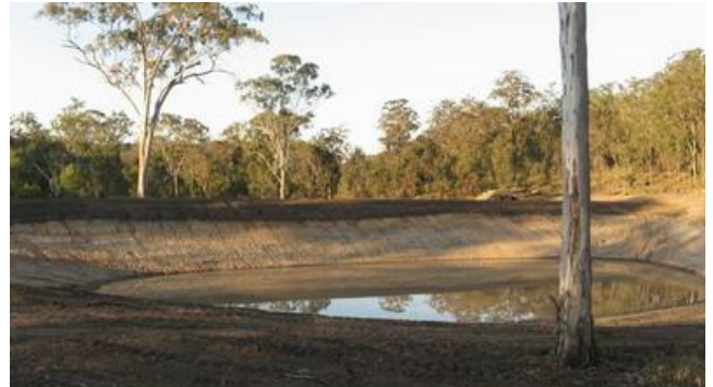
Drowning out a gully head by creating a dam can be a useful way to stabilise a gully.
