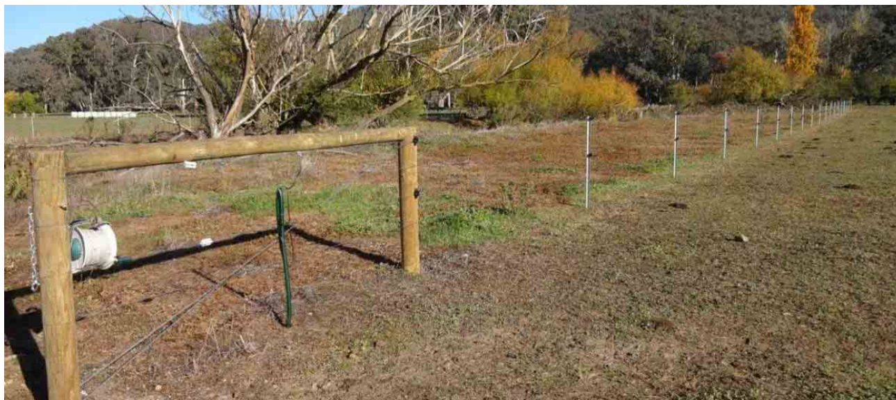
Figure 7.11 – Full-length sacrificial fence
