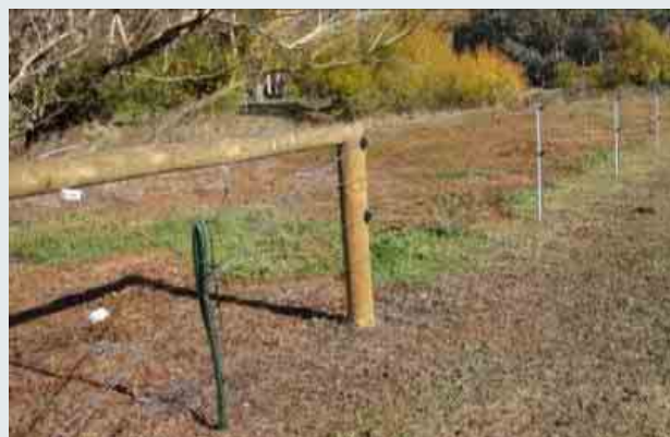
Figure 7.13 – Independent, short sections of fence where flows are expected to be particularly fast, and a point of potential avulsion
