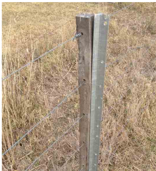
Figure 7.1 – A wooden dropper attached to a star picket
